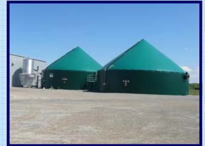
Biogas digesters at Bayview Flowers.
