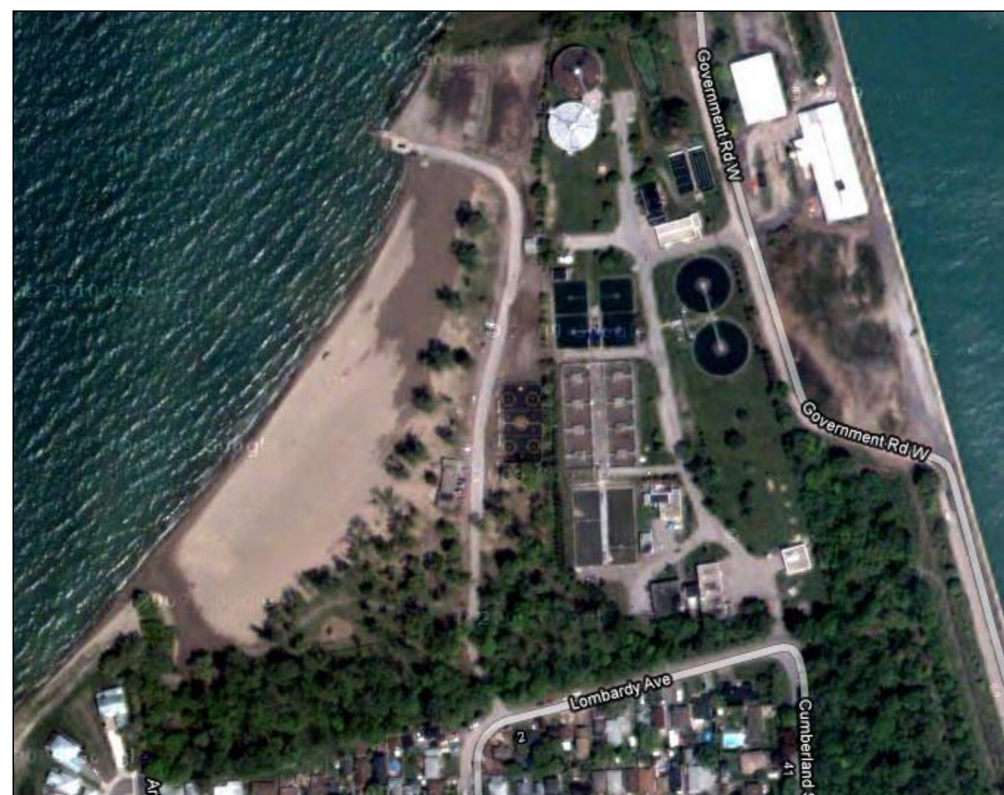
Aerial Photograph of Municipal beach
