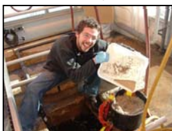
The clearing out of vermiculite and other suspended particles in order to accurately determine the volume of the greenhouse cistern. Continuous water level monitoring data is used to estimate wastewater flow volumes (Gole 2009).
